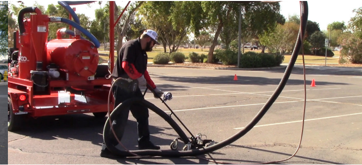
Crack Preparation Equipment
