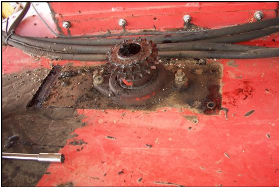
Fig. 6-4 Removal of Motor Mount Assembly
