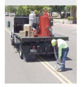
Uniquely formulated with premium ingredients, Crafco's Marker Adhesive remains flexible at temperatures down to 20°F (-7°C) and is specified by several state Departments of Transportation for its remarkable durability. Studies document 50-87% higher marker retention than standard bituminous marker adhesive (Type I) in heavy traffic conditions (>200,000 vehicles daily), with savings from retained markers offsetting any cost differential.
