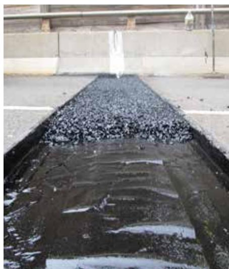
**Transform your bridge joint installation with Matrix 501 – the ultimate solution for flexibility without sacrificing strength.**
