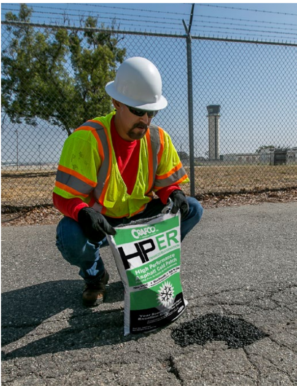
Repaired pothole with High Performance ER Cold Patch.
