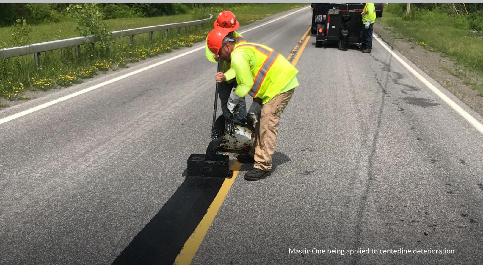
Mastic One being applied to centerline deterioration
