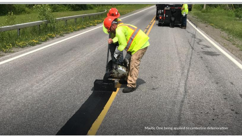
"We have been using Mastic One for about three years," says Rick Jasewicz, a Gorman Group supervisor. "The application was to repair numerous areas of spalling, alligator cracking and potholes. We used this process to repair these areas before a final surface treatment of chip seal was performed."
