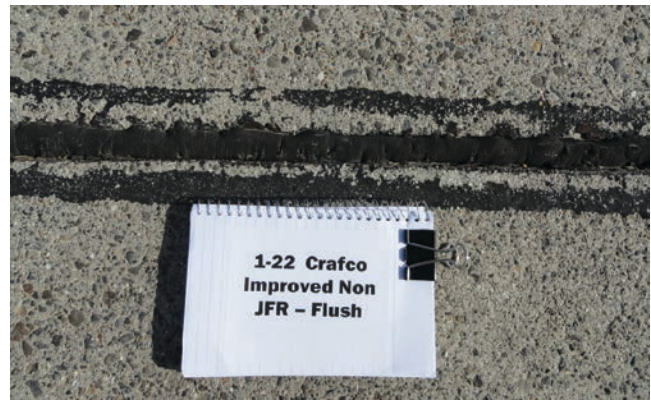
FIGURE 1 Sample of 21-year-old Crafco Improved Non-JFR sealant.
