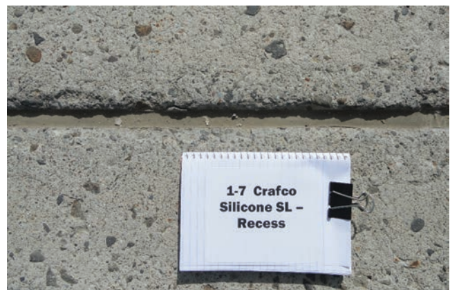
FIGURE 2 Sample of 21-year-old Crafco Silicone SL sealant.
