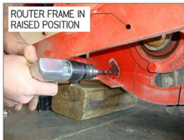
Figure 6-8 Hole Drilling
