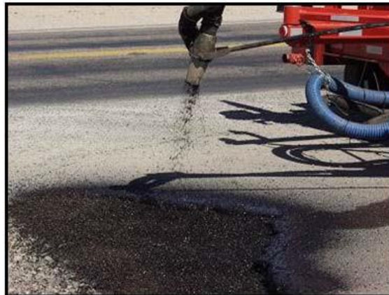
Figure 5.11 Building up the Repair
