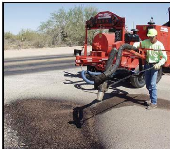
Figure 5.12 Finishing the Repair
