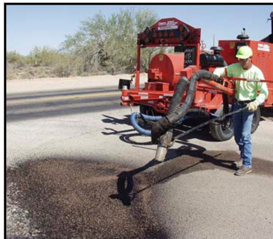
Figure 5.12 Finishing the Repair
