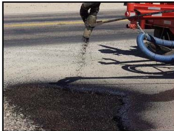
Figure 5.11 Building up the Repair
