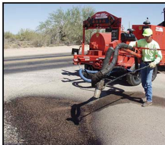
Figure 5.12 Finishing the Repair
