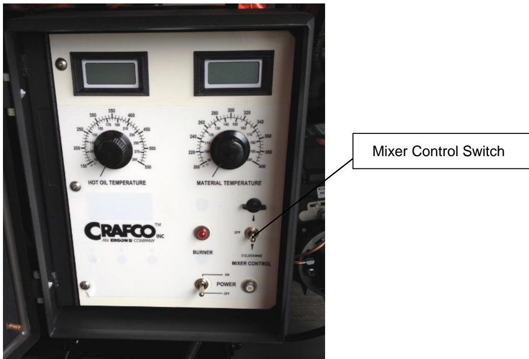
Figure 5.5 Mixer Control Switch
