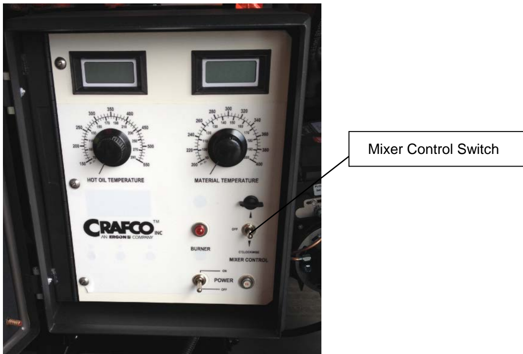
Figure 5.5 Mixer Control Switch
