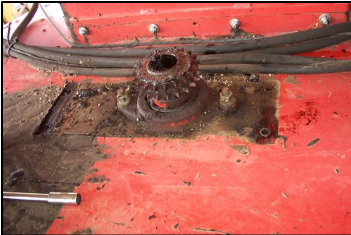
Fig. 6-4 Removal of Motor Mount Assembly
