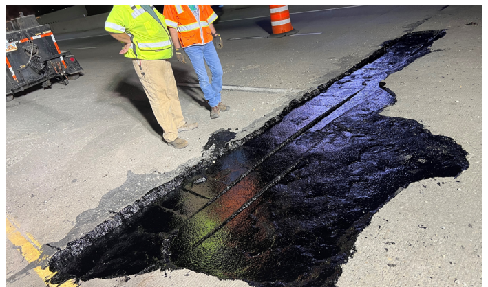
The first lift of Mastic One has been placed and is cooling before next and final lift to be installed. UDOT installed the Mastic One on all edges during the first lift to ensure a waterproof bond on all surface area of the repair.
