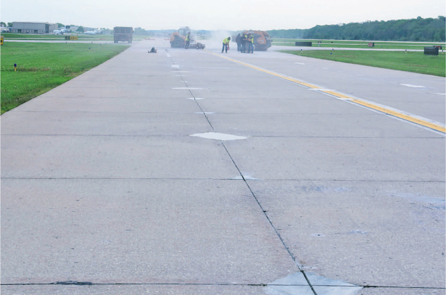
Completed repairs on taxiway using TechCrete.
