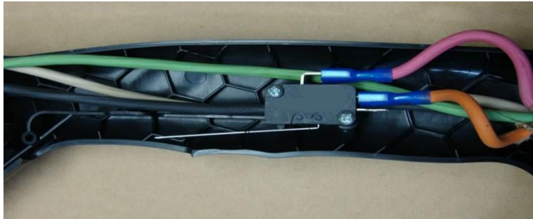
Fig. 6-6 Switch Wire Location
