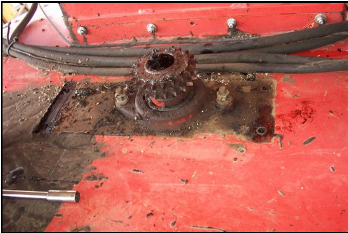
Fig. 6-5 Removal of Motor Mount Assembly
