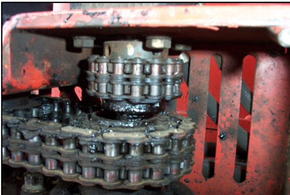
Fig. 6-4 Agitator and Pump Shaft Alignment
