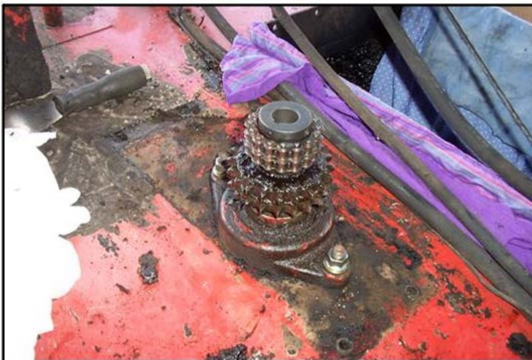
Figure 6.11 Pump Shaft Placement
