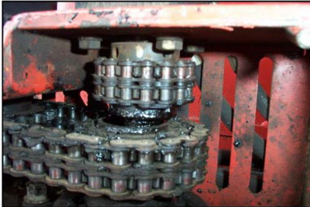
Figure 6.3 Agitator and Pump Shaft Alignment
